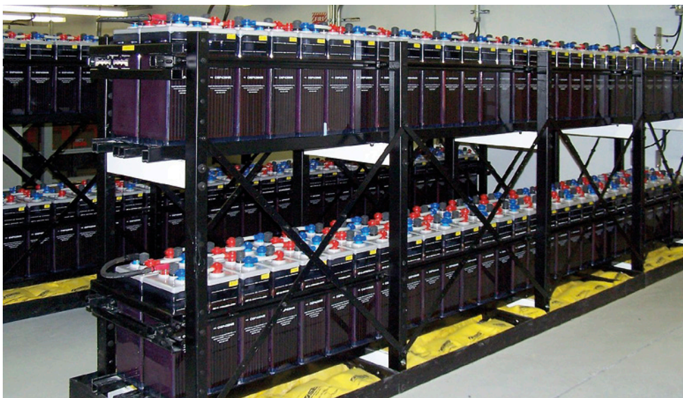
Fig 1: UPS installation series parallel battery connections
